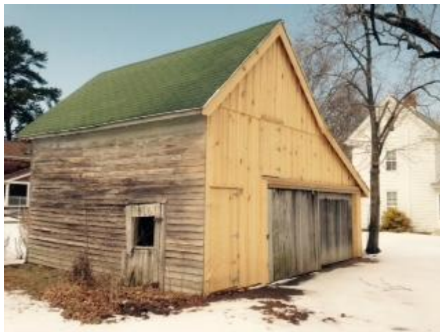
Barn stabilized, not restored
